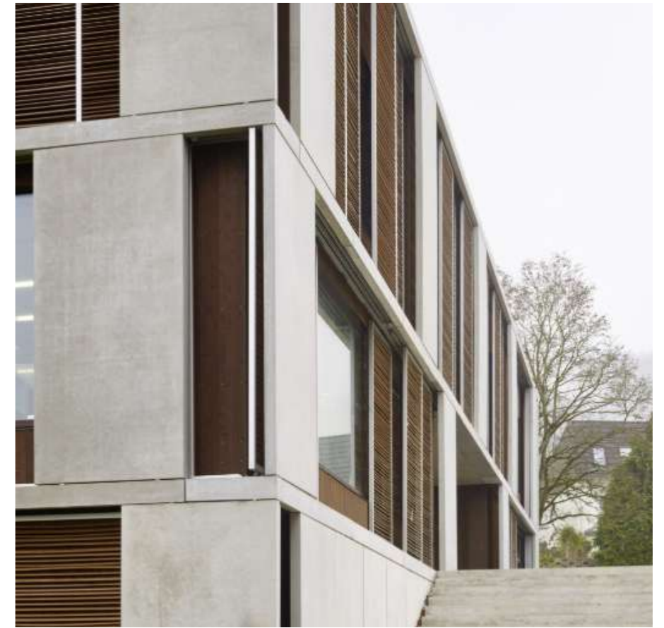
Concrete panels with inset glazing
